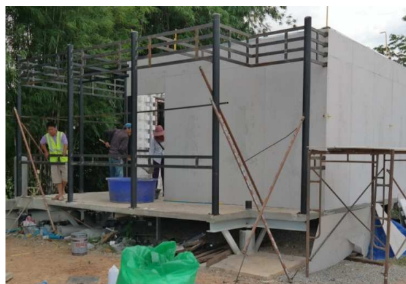
(e) Installation of panels
