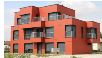
Figure 12: Monitored building from ventilated RAC panels
