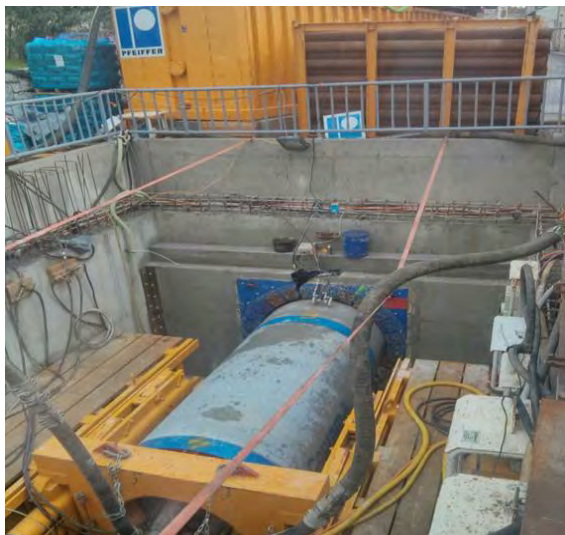
Figure 3. Entrance pit of the microtunnel
