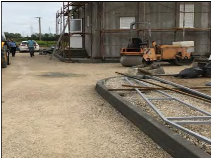
Figure 10. Show placement arrangement of subbase
