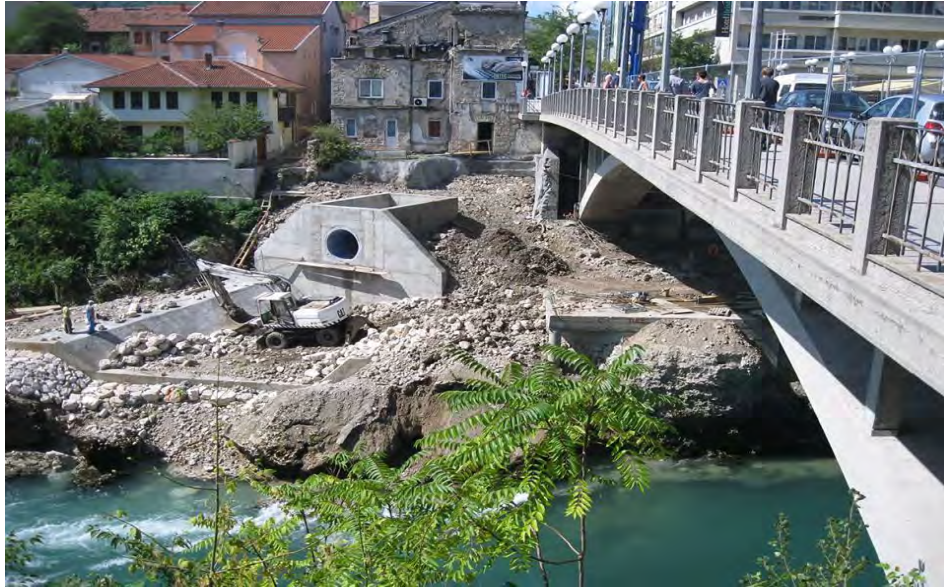
Figure 6. Construction of a stormwater outlet below Tito's Bridge
