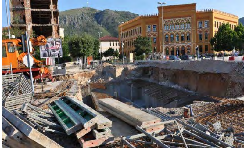
Figure 5. Construction site at the main City Square
