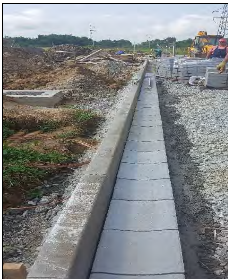
Figure 8. Making concrete channels for the drainage of the road construction
