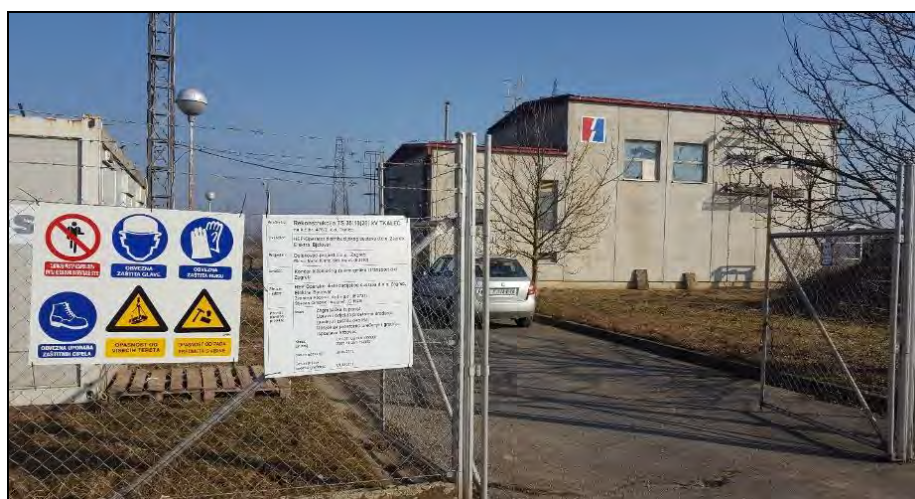
Figure 5. Preparation of construction site TS 35/10 (20) kV Tkalec with a construction board
