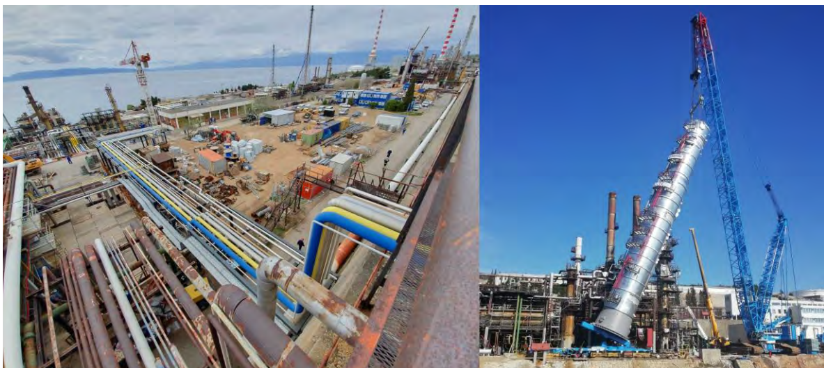
Figure 1. TA of INA Rijeka Refinery 2019 (left) and column assembly – largest CAPEX project (right)
