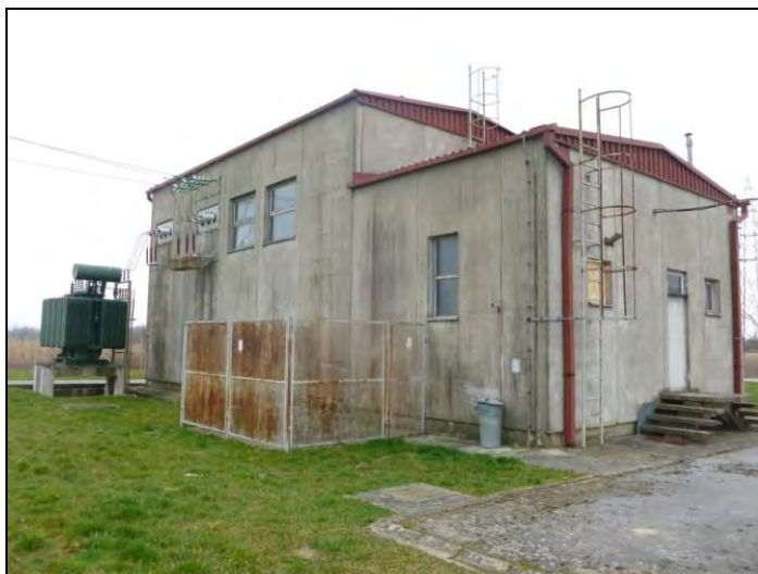
Figure 2. Existing condition of TS 35/10(20) kV Tkalec
