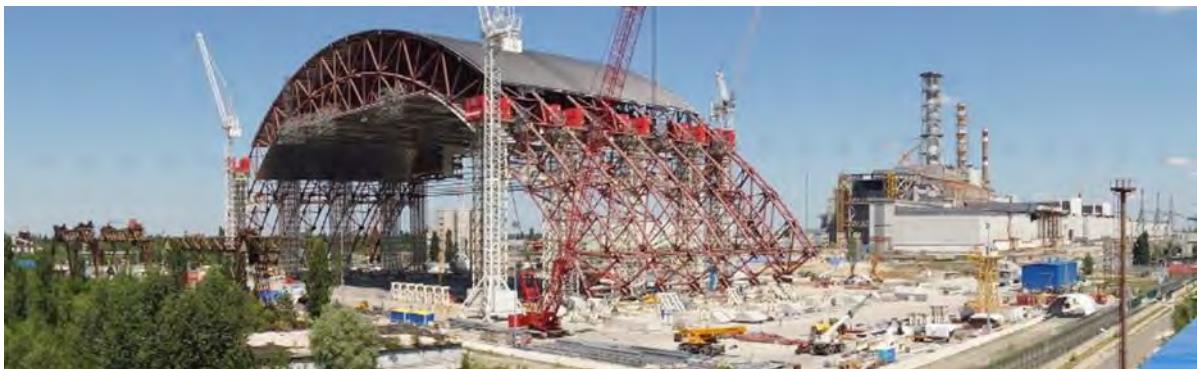
Fig. 2. NSC after the second lift of eastern section in 2013
