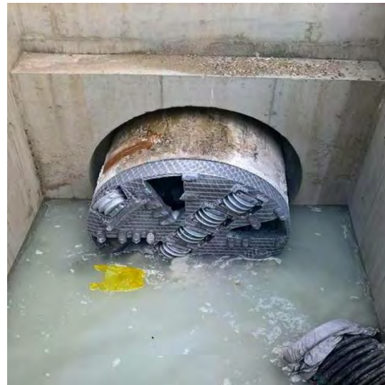
Figure 4. Exit pit of the microtunnel
