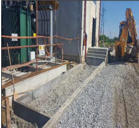
Figure 7. Curb installation along the road
