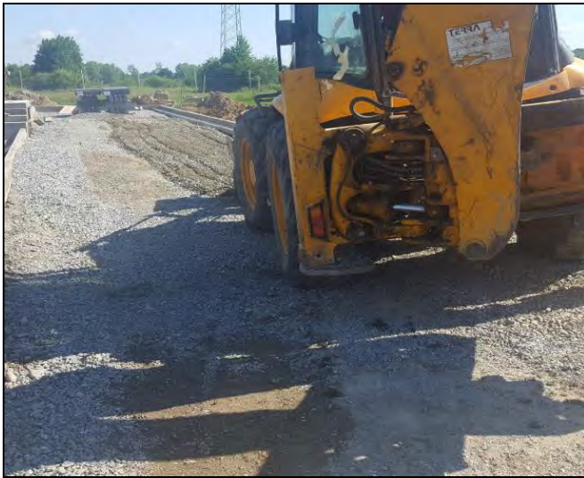
Figure 9. View planning and and profiling of lower layer of the road construction
