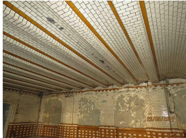
Figure 8: Ceramic tiles in social rooms
