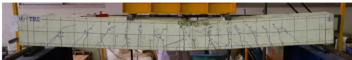
Figure 3: Failure of NSM FRP-strengthened beam TB2
