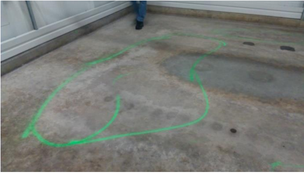
Figure 10: Surface coating spalling
