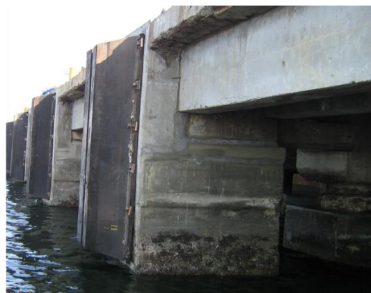
(c) Piers after repair (with rectangular cross-section)
