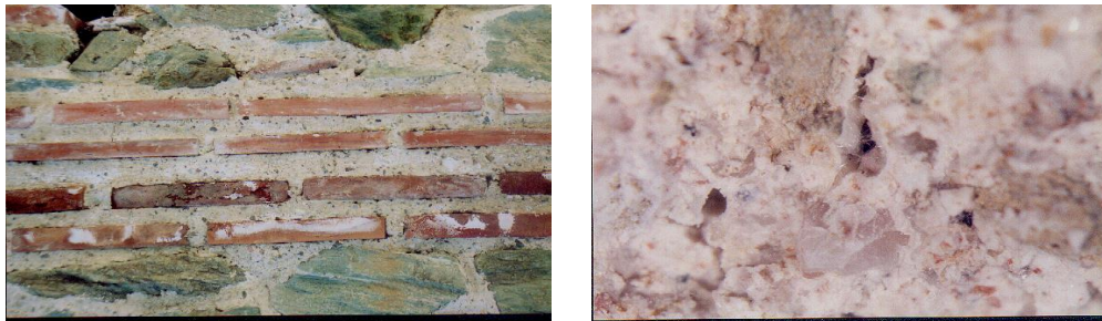
Figure 5: Left: Galerius palace (4 th century BC). Detail of the repaired masonry. Right: Repair mortar from salt damage area of masonry of Galerius Palace. Content in soluble salts which are mostly accumulated into the pores (Cl= 0.28%, NO 3 = 0.83%, SO 4 = 1.14%)
