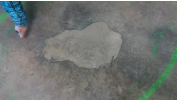
Figure 9: Surface coating spalling
