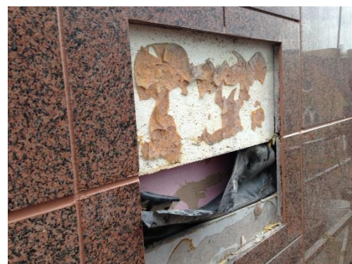
Figure 5 - Details of designed connections and as built connections for granite panels are completely different
