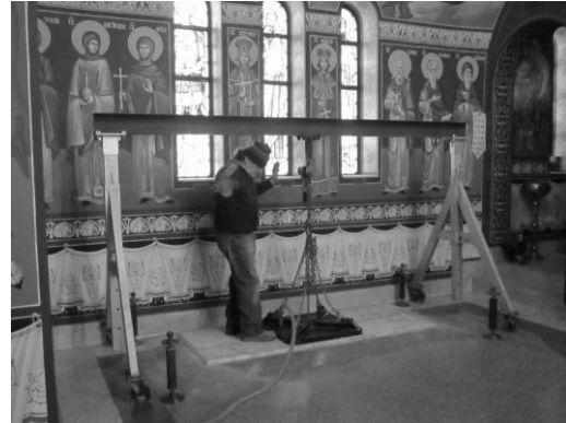
Figure 18: Use of vacuum chamber to lift the stone
