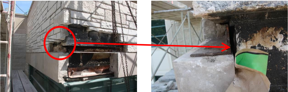
Figure 4 - Overall and close up view of shelf angle detached from structural beam and cracked limestone panel at the back side due to corrosion of shelf angle
