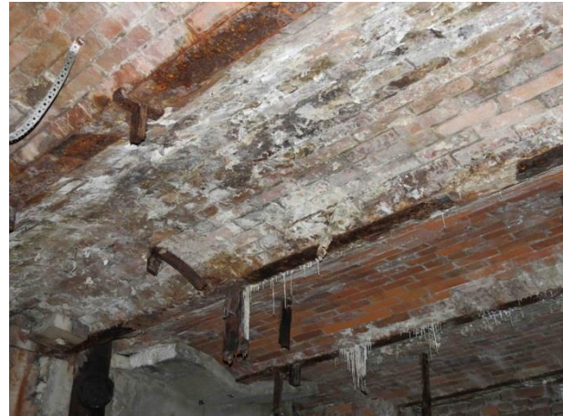
Figure 12: Destruction of brick masonry floors
