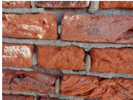
Figure 4: Damage in a trass-lime repointing caused by incomplete hydration of the binding system.
