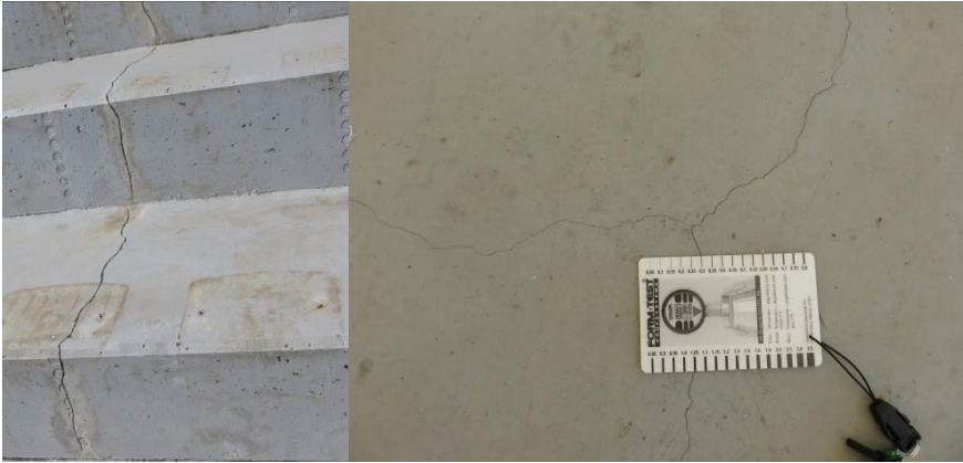
Figure 6: Typical cracks in upper surface
