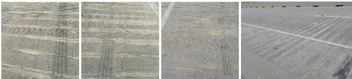
Figure 9: Area repaired after 6 months or traffic. On the two pictures on the left one of the large longitudinal cracks along the beam can be observed being crossed by the FRP strips. No further deterioration was observed since the installation of the NSM FRP strips.
