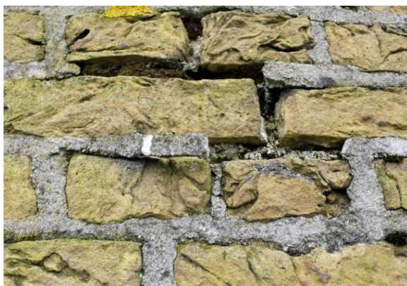
Figure 2: Left: Push out of joints by thermal deformation cycling; Right: graph with E-modulus development of various mortar compositions (NHL mortars, 1:2,5 (vol. parts NHL3,5:sand); cement lime mortars e.g.1:1:6 (vol. parts cement:lime:sand)); (curing conditions 20°C and RH 90%: favourable hydration conditions!)
