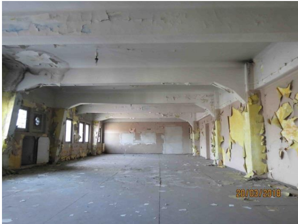
Figure 3: RC structure of the flour warehouse
