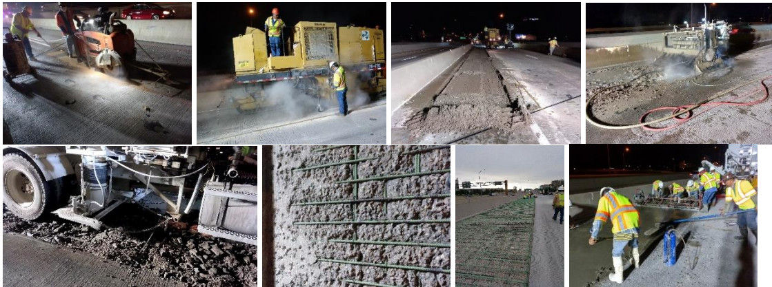
Figure 6: Demolition and reconstruction of overlay – from left to right, top to bottom: Saw cutting of demolition perimeter, milling machine, result of milling, hydrodemolition machine, aspirator truck helping clear debris, left-over rough surface showing original slab, new reinforcement mat in place, and concreting.
