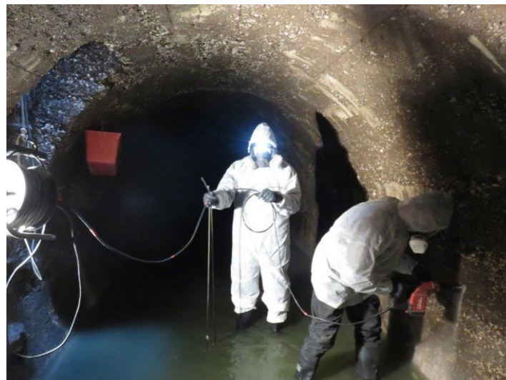
Figure 3: Work conditions inside the sewerage pipe
