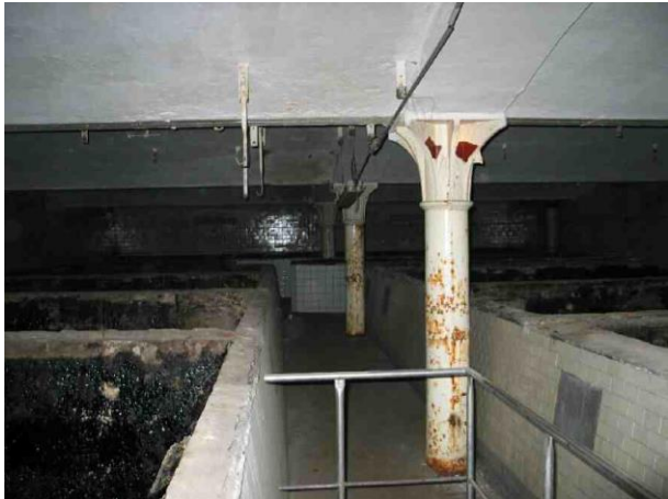
Figure 11: RC reservoirs with cast iron columns
