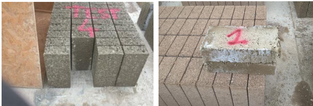
Figure 2. Covered blocks (left) and uncovered blocks with signs of efflorescence (right)
