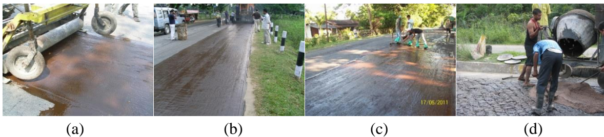
Figure 1: (a) Road in Choygaon; (b) Road towards Airport; (c) Road at Tezpur (d) Microsurfacing over deteriorated plastic cell filled concrete block pavement
