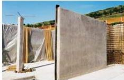
Service Reservoir, England
