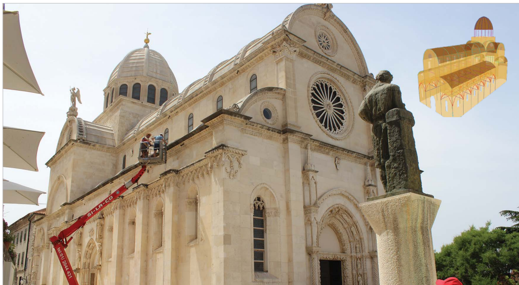
■ SHM system and operational modal analysis of St. Jacobs Cathedral in Šibenik
