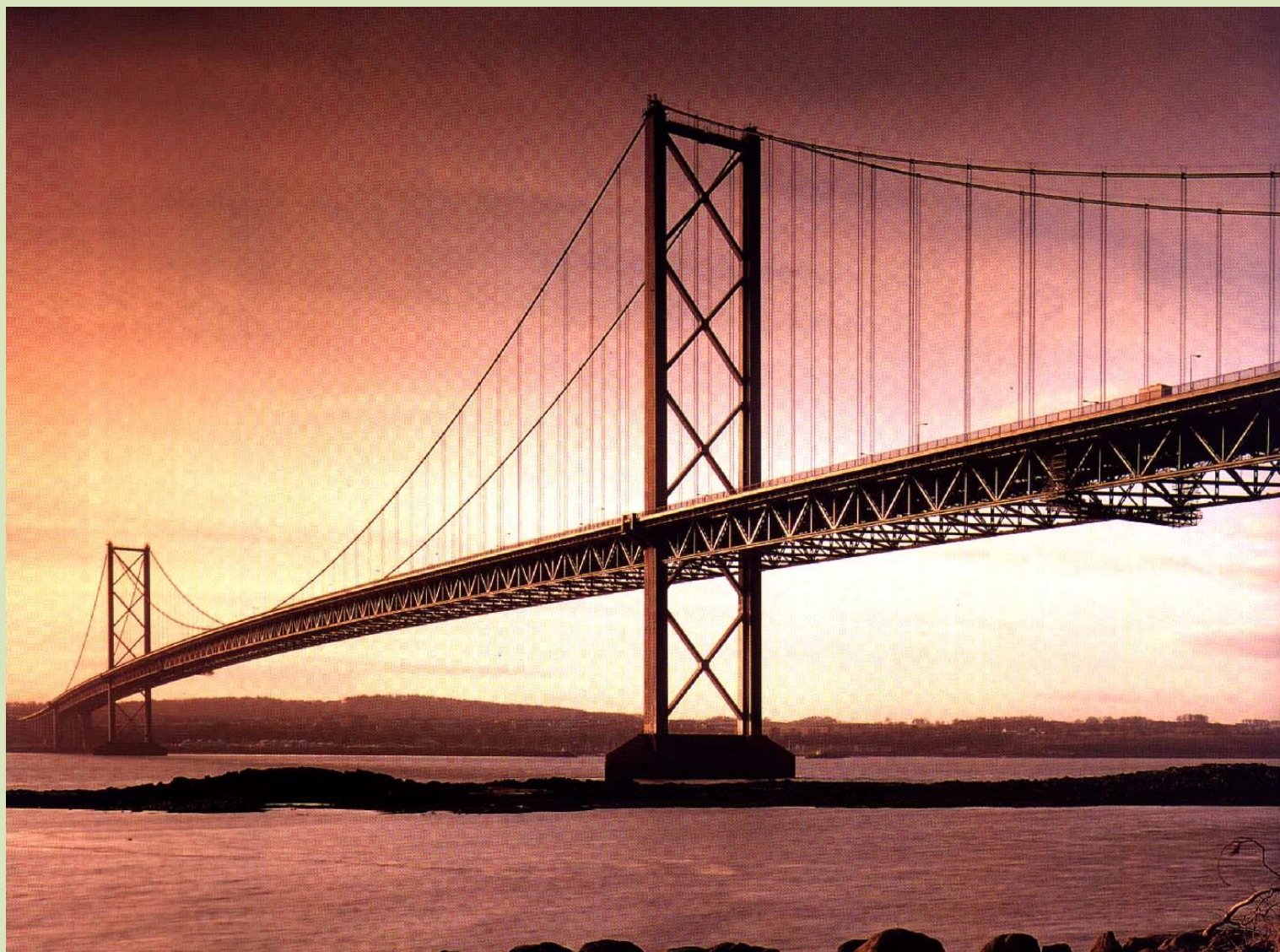
Most Firth of Forth , L=1.064 m, Škotska, 1964.
