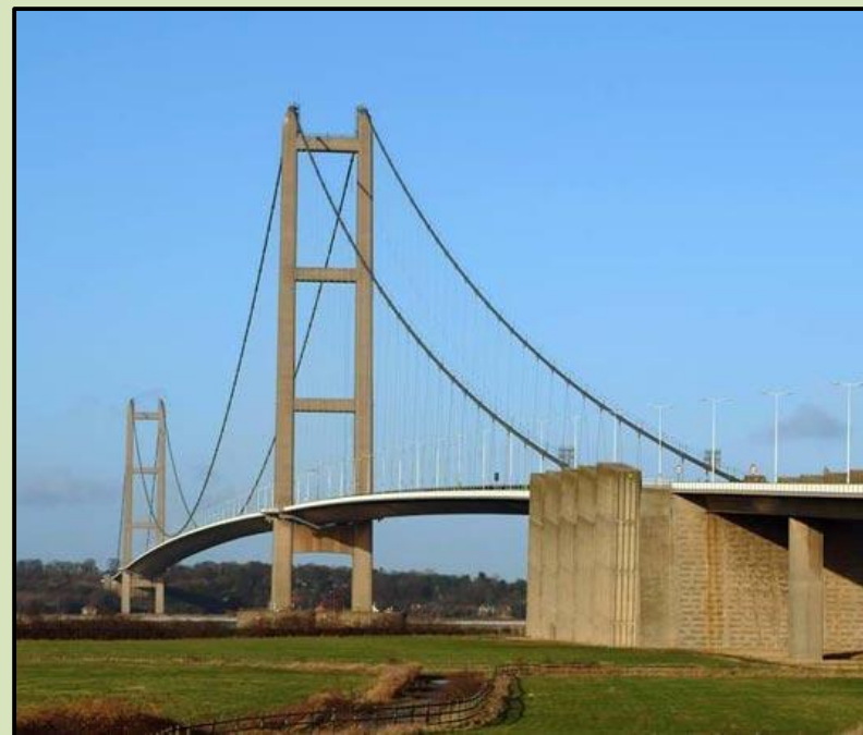
2005., Kina Runyang Bridge, L=1490 m
