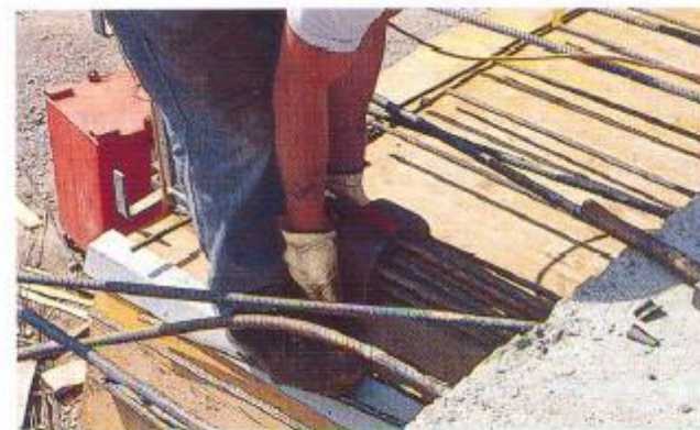
Placing of anchor head
