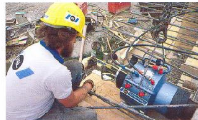
Stressing, measuring, seating of wedges
