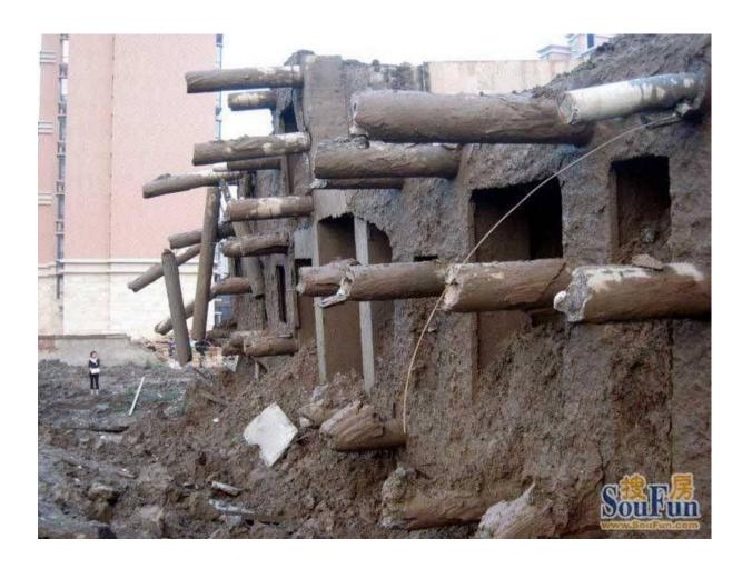
They built 13 stories on grade, with no basement, and tied it all down to hollow pilings with no rebar.
