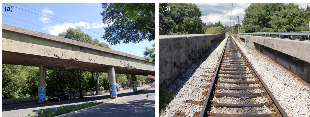
FIGURE 2 Reinforced concrete railway bridge “3. Maj”; (a) side view, (b) top view
