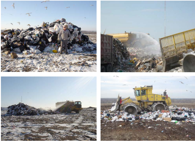
Fig. 1. Photographs of compaction test plot: placement of wastes, water addition to test plot, and compaction
