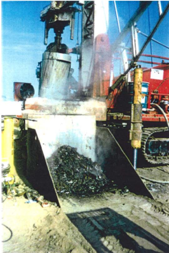
**Fig. 1.** Bucket auger sample recovery at the OII landfill (Geosyntec 1996)
