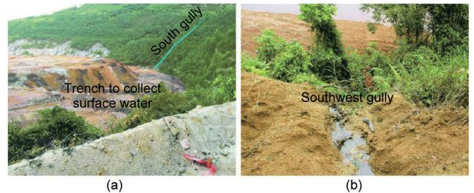
Fig. 16. Gully runoff due to rainfall and continual infiltration to the fresh landfill waste mass at the rear of the landfill. (a) South gully and trench at back, taken on November 24, 2015; (b) permanent discharge of southwest gully to landfill, taken on December 21, 2015.
