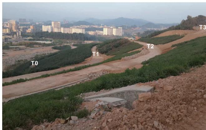
**Fig. 3.** Photograph of the engineered slope and terraces in the front of the landfill taken on October 10, 2015. The surface drainage had been constructed.
