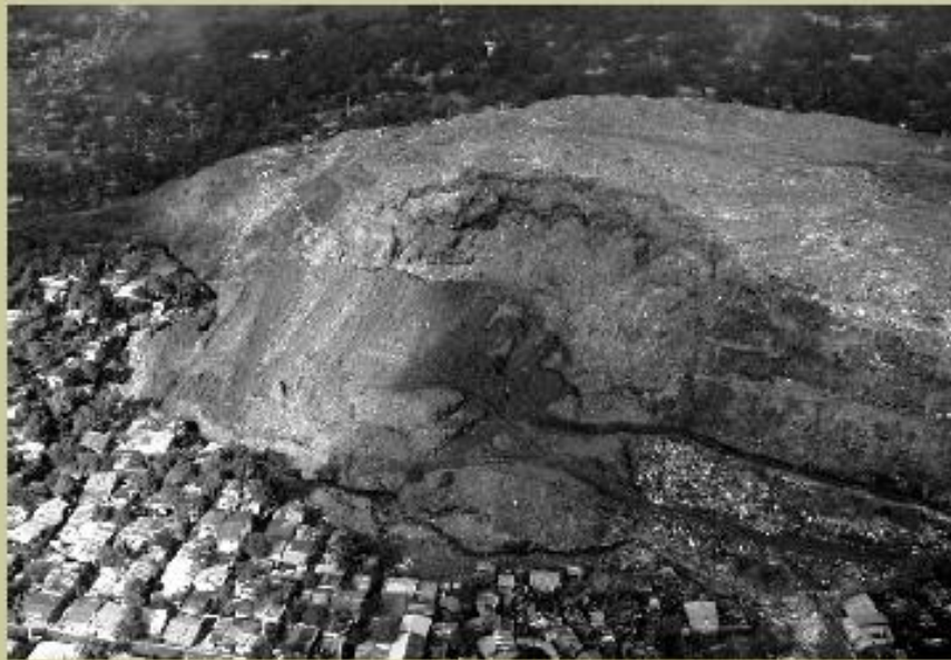
10 July 2000 Payatas Landfill Failure Quezon City, Metropolitan Manila
