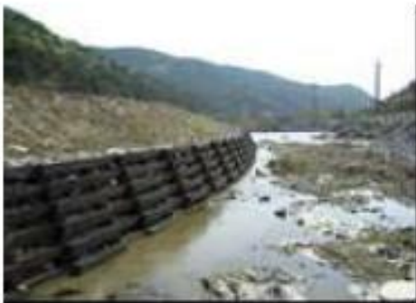
Construction of PE Block
