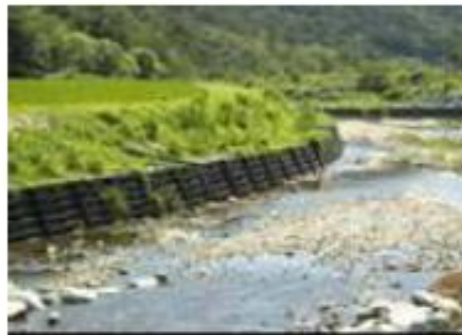
Completion of channel
