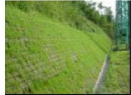
Completion of slope
