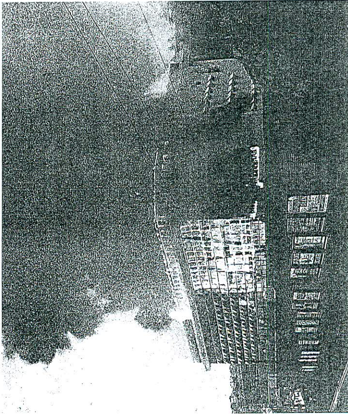
Figure 3.3. Fire spread involving the Oroglas wall and roof of Summerland
