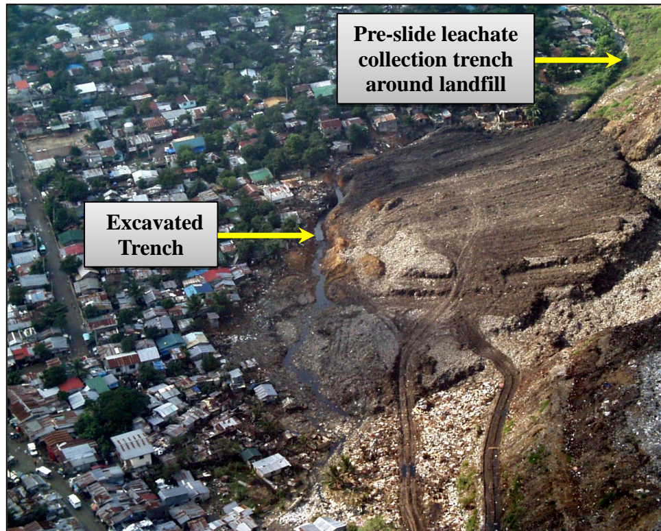
Figure 5. Slope failure showing new and existing leachate trenches along slope toe (photo by S.M. Merry).
