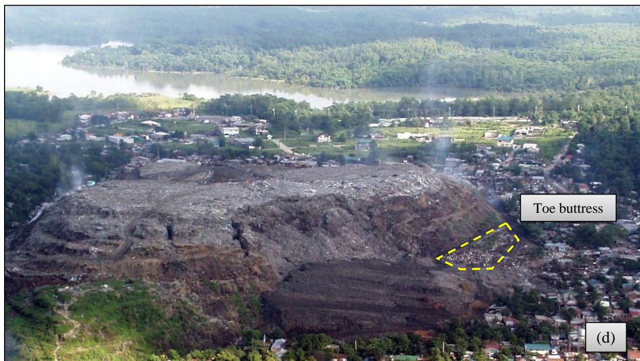
Figure 6. Slope geometry and failure surface after failure (a) evidence of seeping leachate, (b) representative slope inclination, (c) location of slope benches, (d) toe buttress (photos by S.M. Merry).
