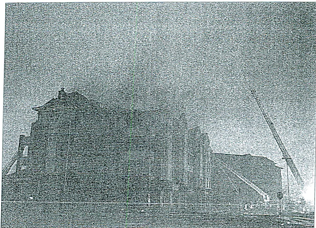
An apartment building suffered $2 million in damage when a leaking propane gas grill on a fourth-floor balcony caused a fire that quickly spread to the roof.
