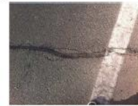
Bjelovar bridge: repaired asphalt pavement cracks; concrete cover fraction and reinforcing steel corrosion at the superstructure slab bottom; soil erosion at the embankment cone
