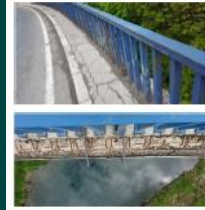
Rastoke bridge: corrosion protection decline of the pedestrian fence; concrete cover fracture and reinforcing steel corrosion of the cornice; concrete cover delamination and efflorescence at the slab bottom; segregation and reinforcing steel corrosion at the bottom slab next to the abutment
