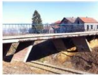
Bjelovar bridge: repaired asphalt pavement cracks; concrete cover fraction and reinforcing steel corrosion at the superstructure slab bottom; soil erosion at the embankment cone
