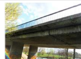
Korana bridge: mechanical damage and corrosion of pedestrian fence; asphalt pavement cracks and dilatation related to expansion joint; dilatation, concrete wetting and efflorescence at the main slab girders; cornice delamination
