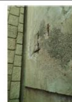
Rastoke bridge: corrosion protection decline of the pedestrian fence; concrete cover fracture and reinforcing steel corrosion of the cornice; concrete cover delamination and efflorescence at the slab bottom; segregation and reinforcing steel corrosion at the bottom slab next to the abutment
