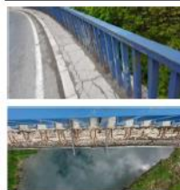
Rastoke bridge: corrosion protection decline of the pedestrian fence; concrete cover fracture and reinforcing steel corrosion of the cornice; concrete cover delamination and efflorescence at the slab bottom; segregation and reinforcing steel corrosion at the bottom slab next to the abutment
