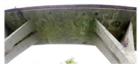
Rastoke bridge: corrosion protection decline of the pedestrian fence; concrete cover fracture and reinforcing steel corrosion of the cornice; concrete cover delamination and efflorescence at the slab bottom; segregation and reinforcing steel corrosion at the bottom slab next to the abutment
