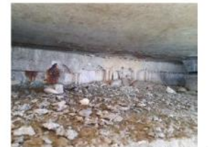
Gradna bridge: corrosion of pedestrian fence; side walk mix routing and curb erosion; cornice wetting; wetting and delamination of concrete of the pier; leaking, wetting and delamination at the abutment
