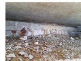
Gradna bridge: corrosion of pedestrian fence; side walk mix routing and curb erosion; cornice wetting; wetting and delamination of concrete of the pier; leaking, wetting and delamination at the abutment
