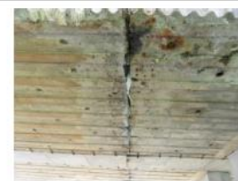
Korana bridge: mechanical damage and corrosion of pedestrian fence; asphalt pavement cracks and dilatation related to expansion joint; dilatation, concrete wetting and efflorescence at the main slab girders; cornice delamination
