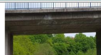
Slunjčica bridge: concrete cover fraction and reinforcing steel corrosion at the pier; and at the slab bottom; sidewalk block cracking, mix rutting and asphalt crack at the pavement
