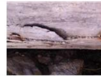
Bjelovar bridge: repaired asphalt pavement cracks; concrete cover fraction and reinforcing steel corrosion at the superstructure slab bottom; soil erosion at the embankment cone
