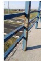
Gradna bridge: corrosion of pedestrian fence; side walk mix routing and curb erosion; cornice wetting; wetting and delamination of concrete of the pier; leaking, wetting and delamination at the abutment
