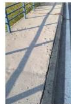
Gradna bridge: corrosion of pedestrian fence; side walk mix routing and curb erosion; cornice wetting; wetting and delamination of concrete of the pier; leaking, wetting and delamination at the abutment
