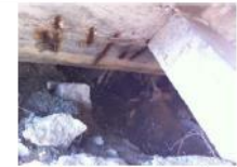
Bjelovar bridge: repaired asphalt pavement cracks; concrete cover fraction and reinforcing steel corrosion at the superstructure slab bottom; soil erosion at the embankment cone
