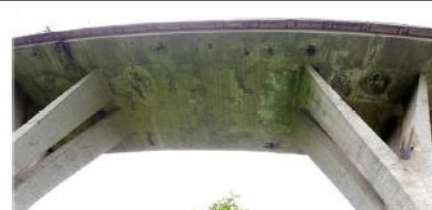
Rastoke bridge: corrosion protection decline of the pedestrian fence; concrete cover fracture and reinforcing steel corrosion of the cornice; concrete cover delamination and efflorescence at the slab bottom; segregation and reinforcing steel corrosion at the bottom slab next to the abutment
