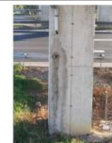
Gradna bridge: corrosion of pedestrian fence; side walk mix routing and curb erosion; cornice wetting; wetting and delamination of concrete of the pier; leaking, wetting and delamination at the abutment
