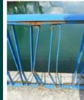
Korana bridge: mechanical damage and corrosion of pedestrian fence; asphalt pavement cracks and dilatation related to expansion joint; dilatation, concrete wetting and efflorescence at the main slab girders; cornice delamination
