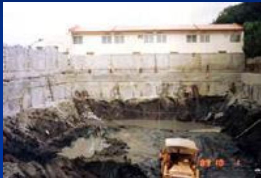
Iskop s bermom
