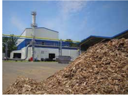
Wood biomass power plant
