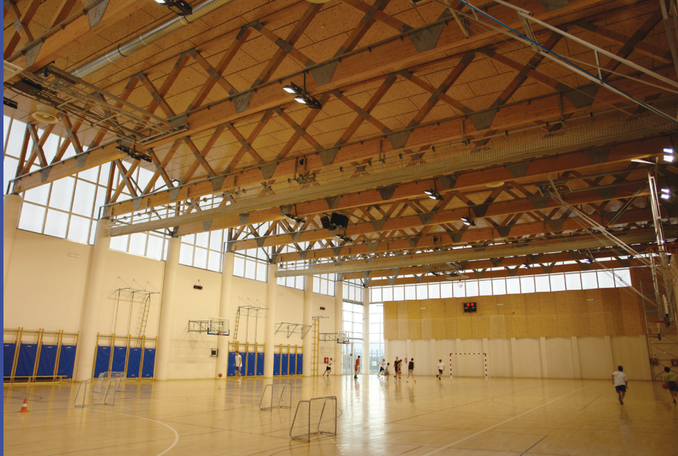
— Timber truss roof structure of the Crafts school and City of Samobor sport hall
